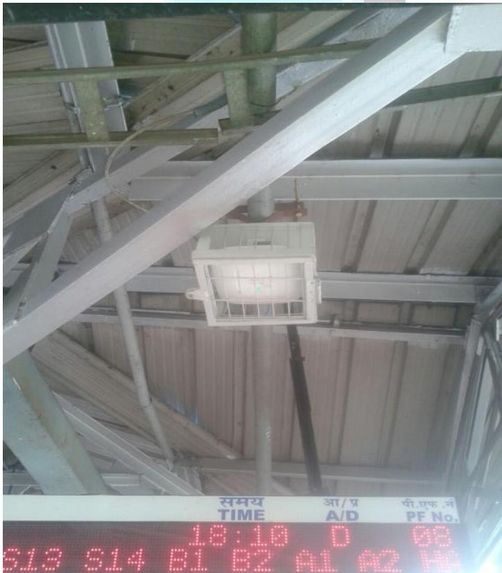
A model Photograph of Rack and Access point metal cage installation at Railway station FOB/Platform shed , but as per the site condition to be installed with all accessories
