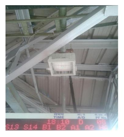
A model Photograph of Rack and Access point metal cage installation at Railway station FOB/Platform roof as per the site condition to be installed with all accessories.
