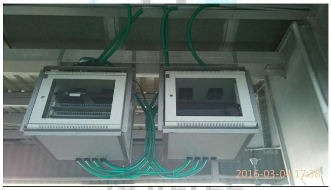
Photograph of Rack( installation )at Railway station FOB/Platform shed as per site condition and as per Instruction of section/site in charge. Installation includes supply of material and proper fixture required for installation as per Railway standard.
